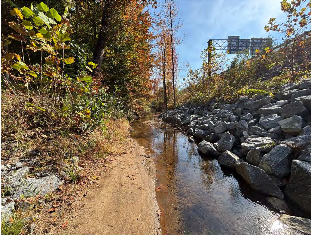
Looking Downstream at Transition Zone Streambank Repairs – November 2025
