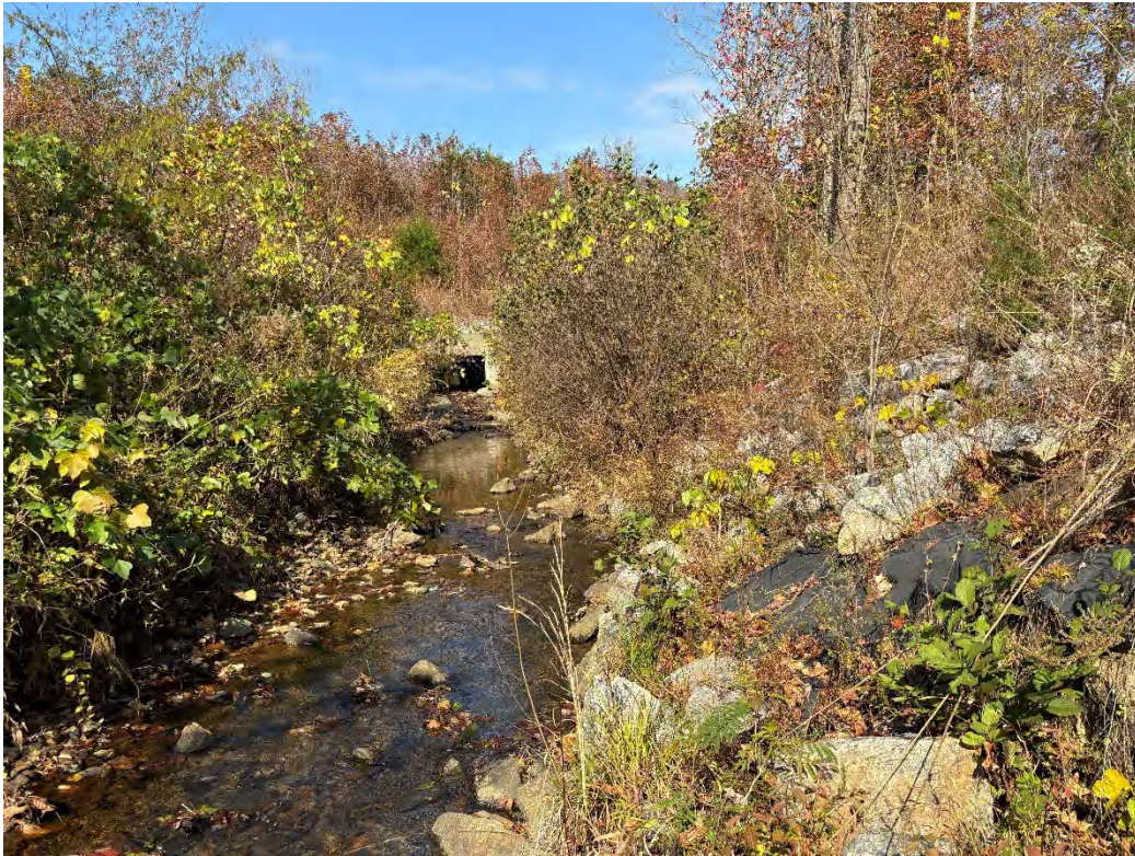
Looking Upstream toward RCBC – Beginning of Channel Change – North End
