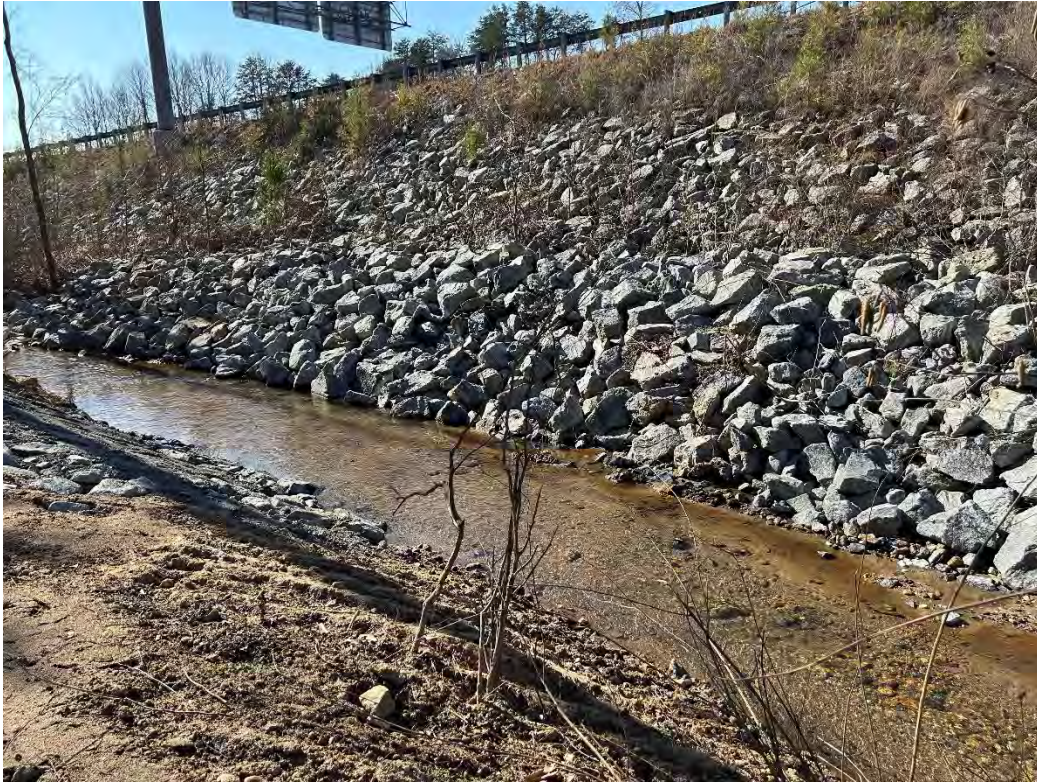
Transition Zone Streambank Repairs Completed February 2025
