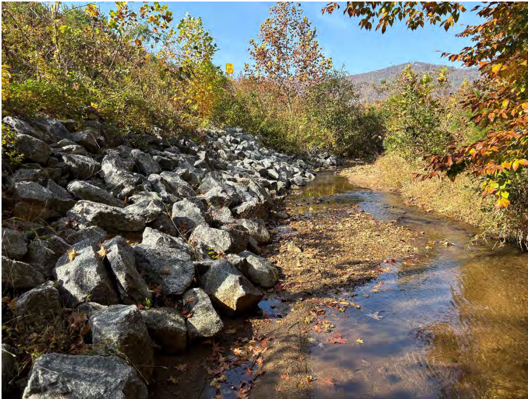
Looking Upstream at Transition Zone Streambank Repairs – November 2025
