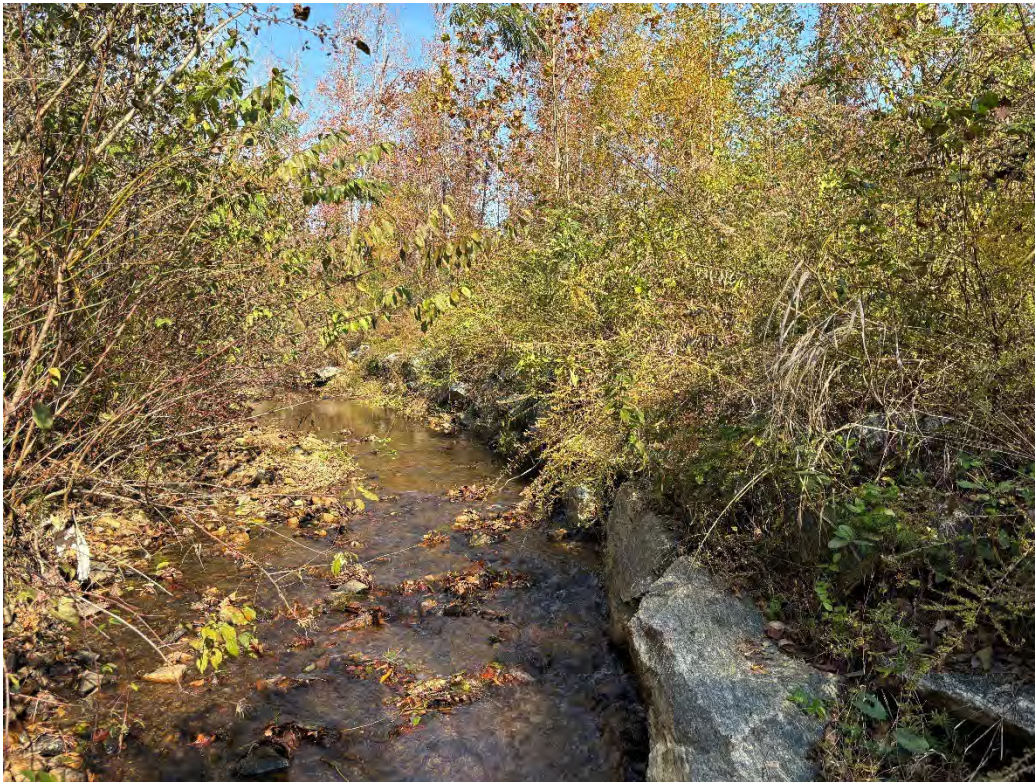
Looking Upstream at Shot Rock Bank Stabilization Repairs from 2020
